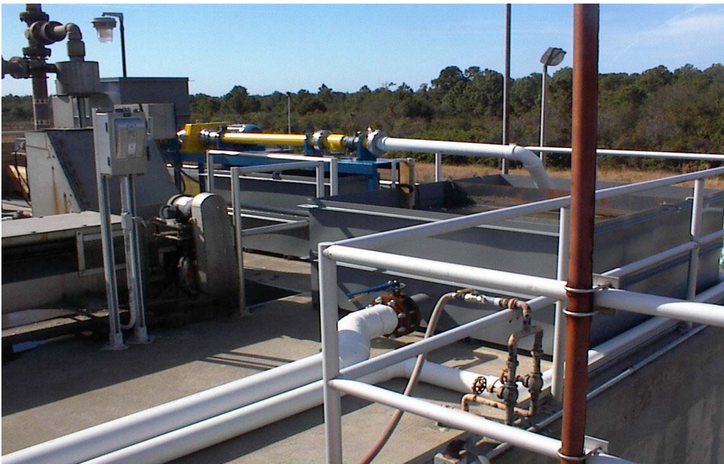
Figure 4 - View of Voraxial™ Grit Separator, Grit Collector Tank and Main Tank
