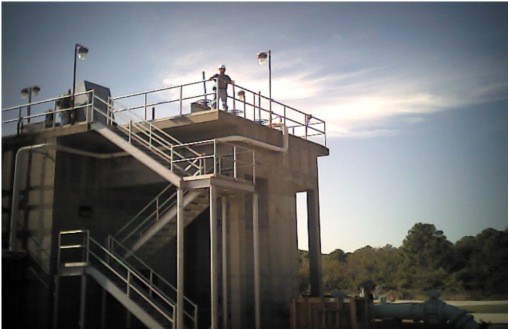
Figure 2 - Northwest Regional Water Reclamation Facility Headworks
