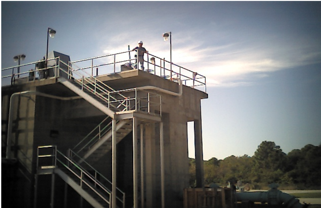
Figure 2 - Northwest Regional Water Reclamation Facility Headworks
